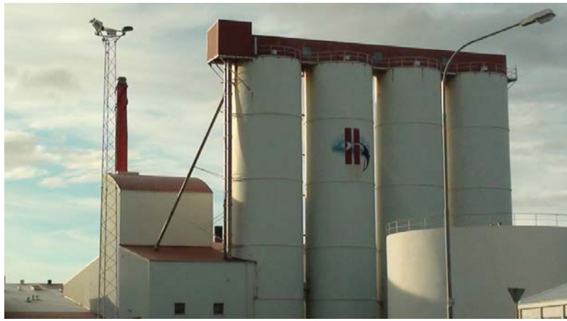
© WDCS ABOVE: HB Grandi fish meal silos, Akranes.
