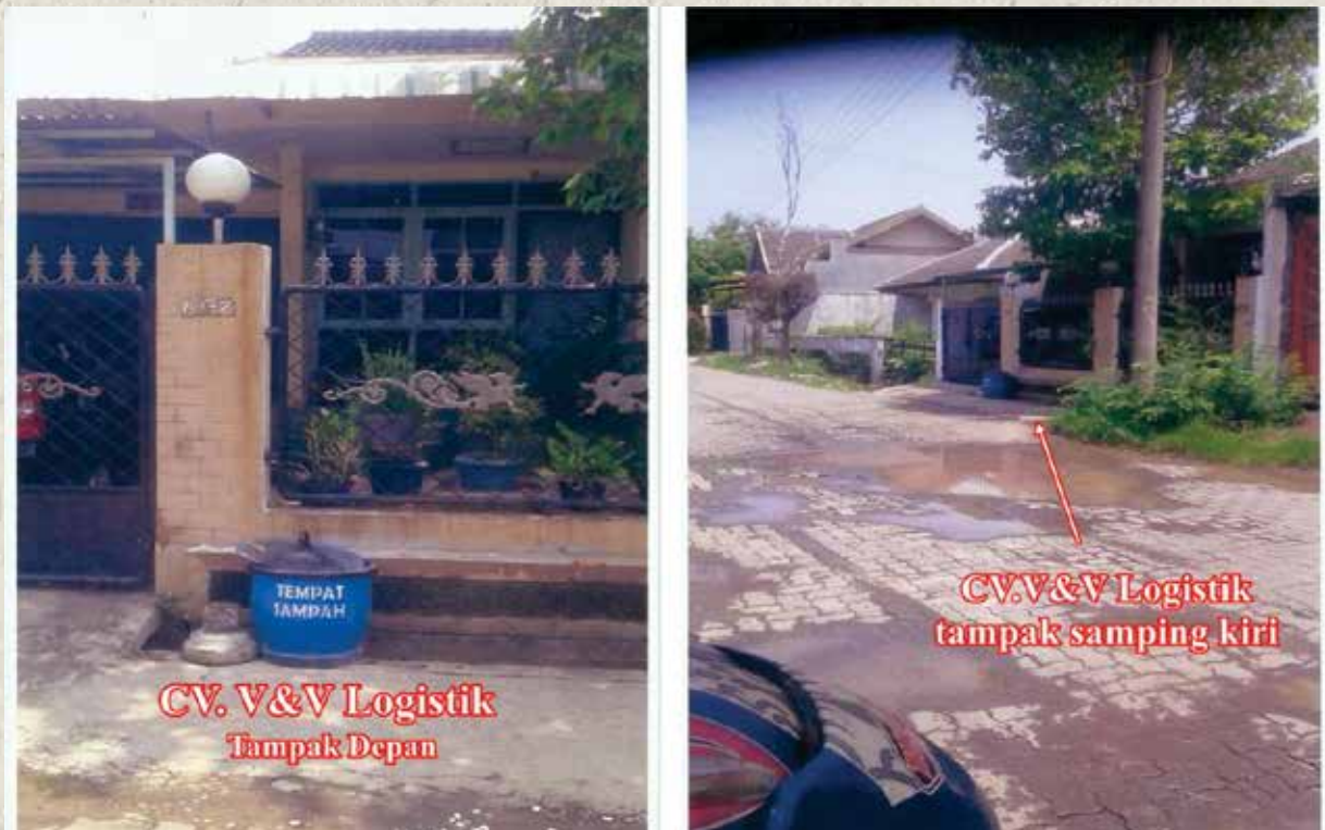
Figure 1. CV V&V location and logistics facilities.
