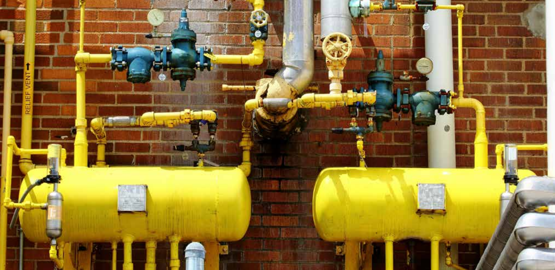
Above: Ammonia refrigeration piping and tanks
