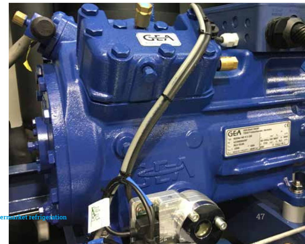
Below: GEA's CO 2 compressor
