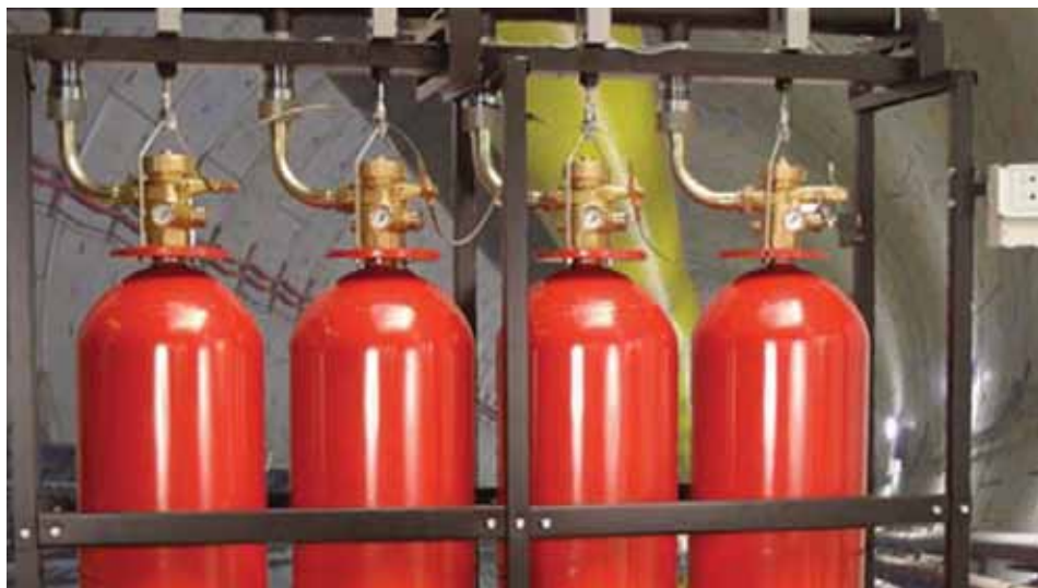
FE-13TM (HFC-23) fire extinguishing agent is the product of Dupont. Dupont and other companies in the EU, US and China are selling HFC-23 for fire suppression systems rather than destroying it despite the availability of low/zero ODP/GWP alternatives.
