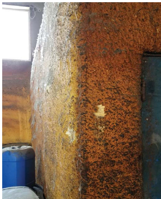
Wall containing foam produced in Dacheng Desheng Chemical Co., Ltd, holes poked to showcase strength of foam by factory representative
