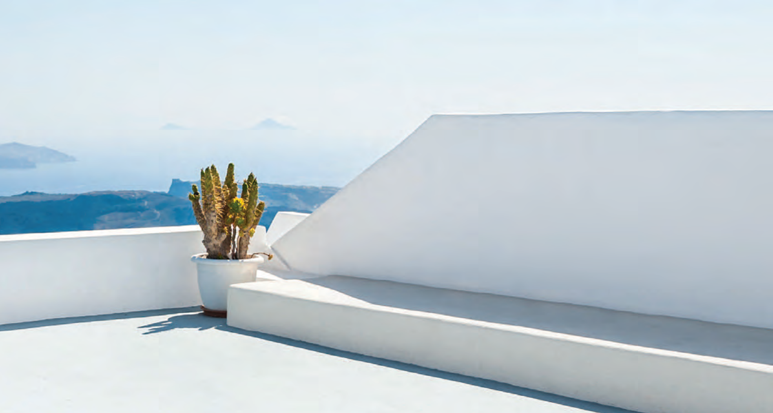
Above: A cool roof painted white to reflect sunlight and absorb less heat.
